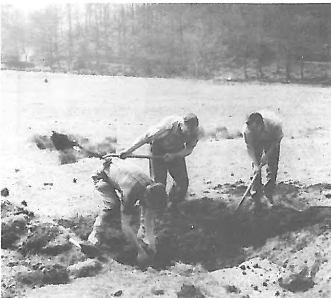
Above: Work commences on the installation of the septic tank summer 1958
